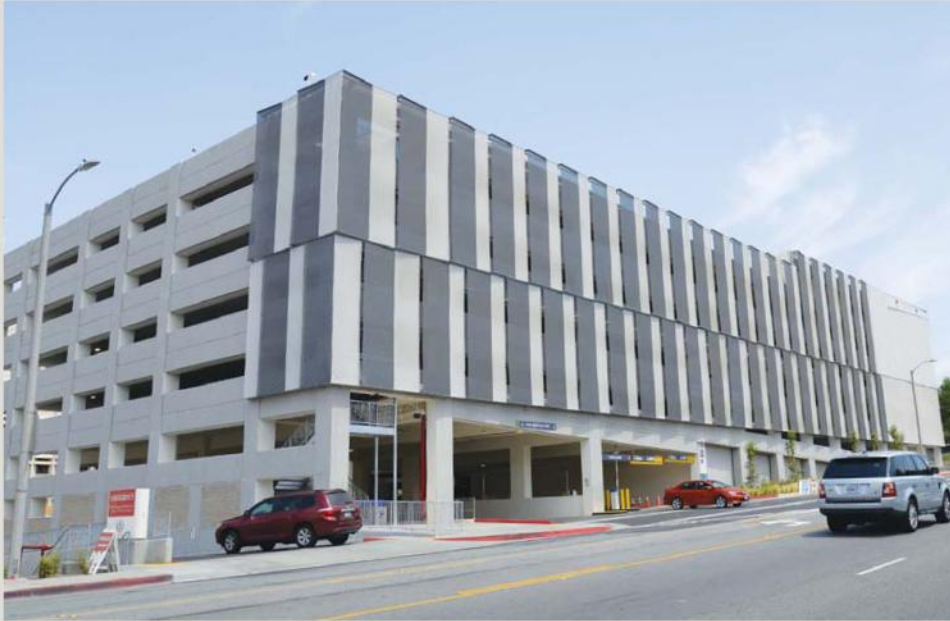
At the Loma Linda University carpark in San Bernardino, California, Kaynemaile-Armour mesh has been fashioned into louvre-like strips that significantly mitigate the area's hot, dry conditions.
