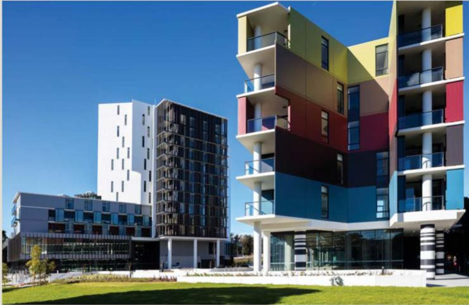
Taubmans Armawall Armashield coats the fibre cement sheeting and precast concrete external walls to ensure long-term durability, while cladding and balcony blades on the Epsom Road building are finished in Taubmans All Weather Low Sheen water-based paint – both feature dirt-shedding technology.
